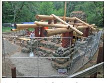
Bear Hut at Natalie Coffin Greene Park. Because of the historical significance of the structure, the structure is being rebuilt utilizing as much of the original wood material as possible. All of the log components of the structure have been either repaired or milled from newer redwood and the hut is being reassembled using some of the same hand work and techniques used
