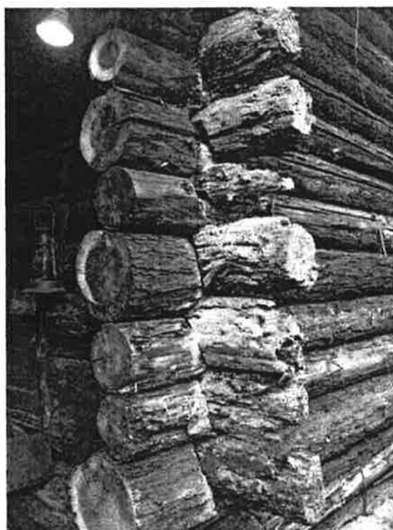
Photo 5. Northwest corner of cabin, showing deteriorated log ends. (Carey & Co. November, 2006)
