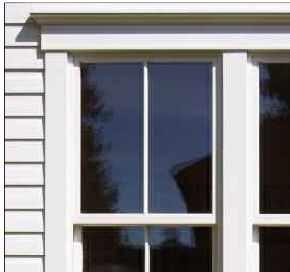
PAINTED WOOD WINDOWS AND DOORS WHITE
