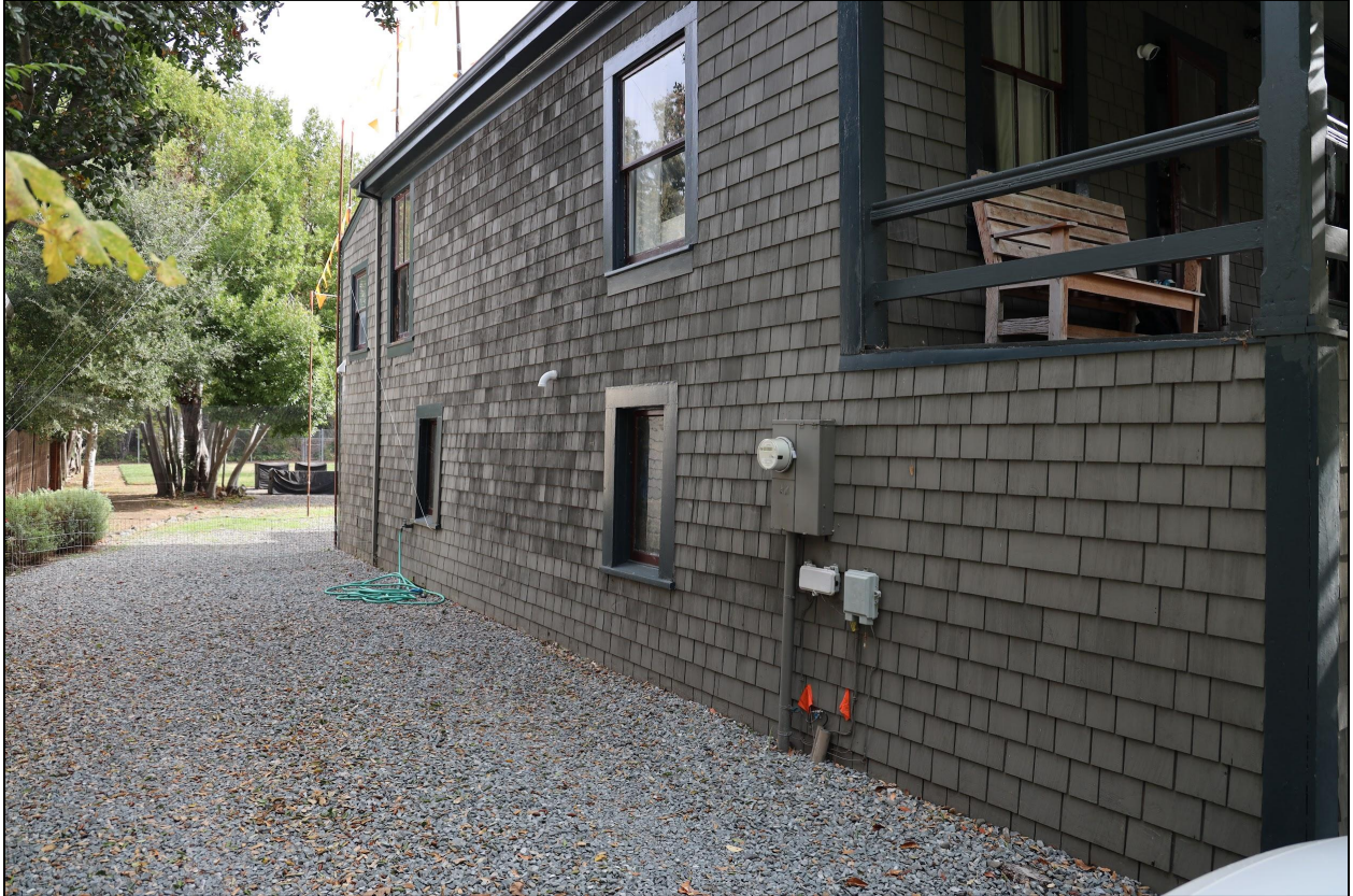
North facade, 45 Poplar Avenue, November 2023 (Source: Watson Heritage Consulting)
