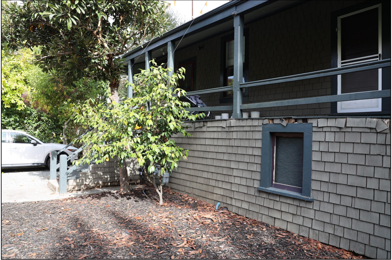
Entrance porch, west facade, 45 Poplar Avenue, November 2023 (Source: Watson Heritage Consulting)
