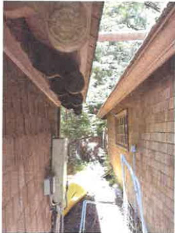
VIEW OF NORTH SIDE OF GARAGE, POOL EQ ON LEFT
