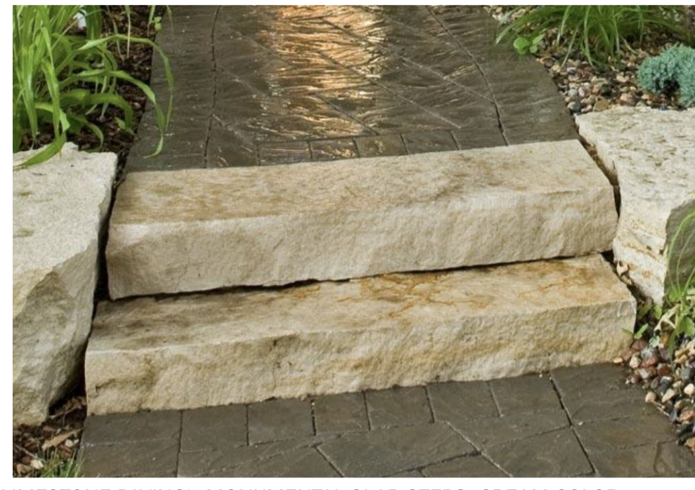
B, C BRICK CHEEK WALLS WITH LIMESTONE CAP (MATCH LIMESTONE PAVING); MONUMENTAL SLAB STEPS, CREAM COLOR
