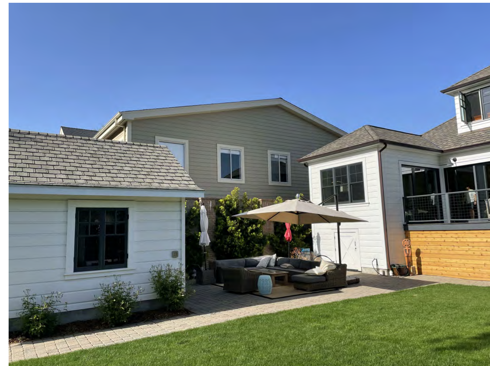
32 POPLAR FROM 34 POPLAR YARD
