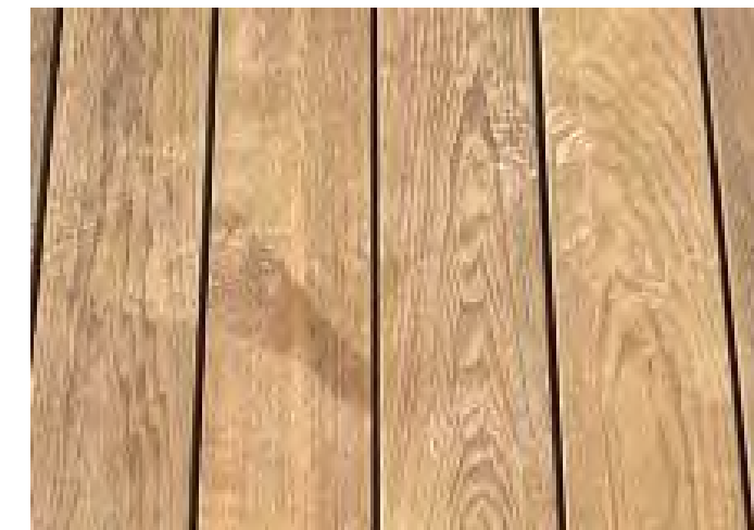
DECK AT ADU ENTRY: THERMALLY MODIFIED WOOD THERMORY ASH OR EQUAL
