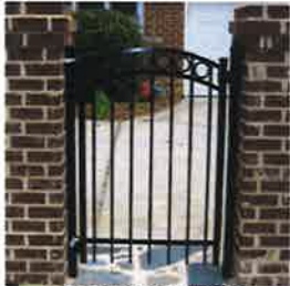
IRON PEDESTRIAN GATE
