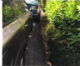
4 CURRENT GUTTER/GUEST PARKING
