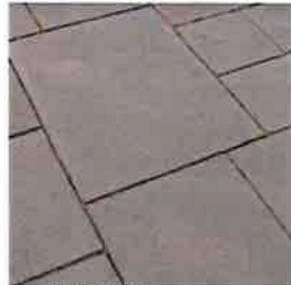
BLUESTONE PAVING ON PERMEABLE BASE
