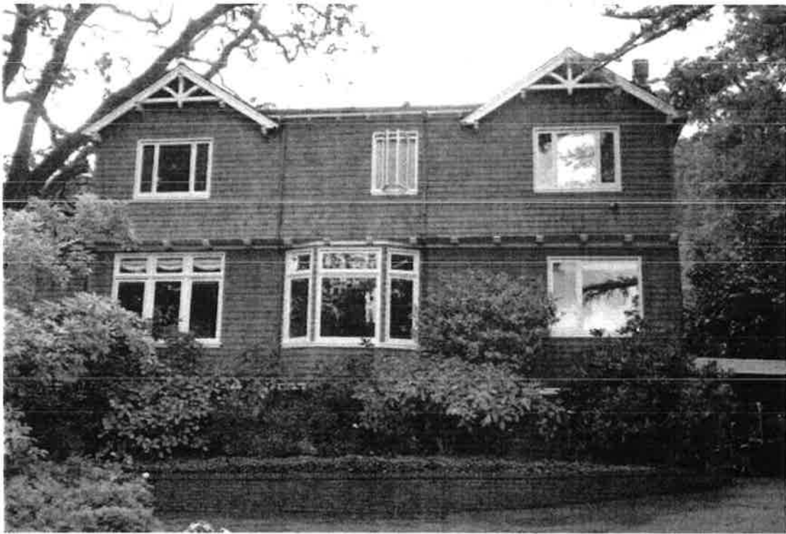
Fig.5 – 147 Lagunitas Rd. – Front (north) facade (2014)
