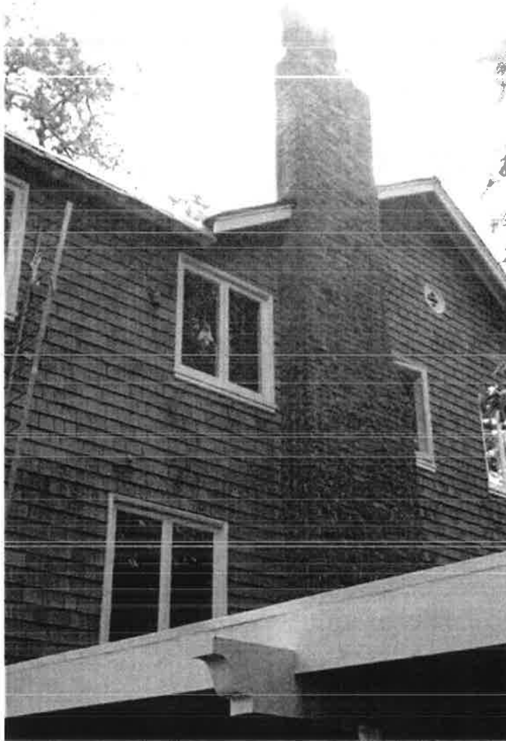
Fig.7 – 147 Lagunitas Rd. – West side with older carport roof in foreground (2014)
