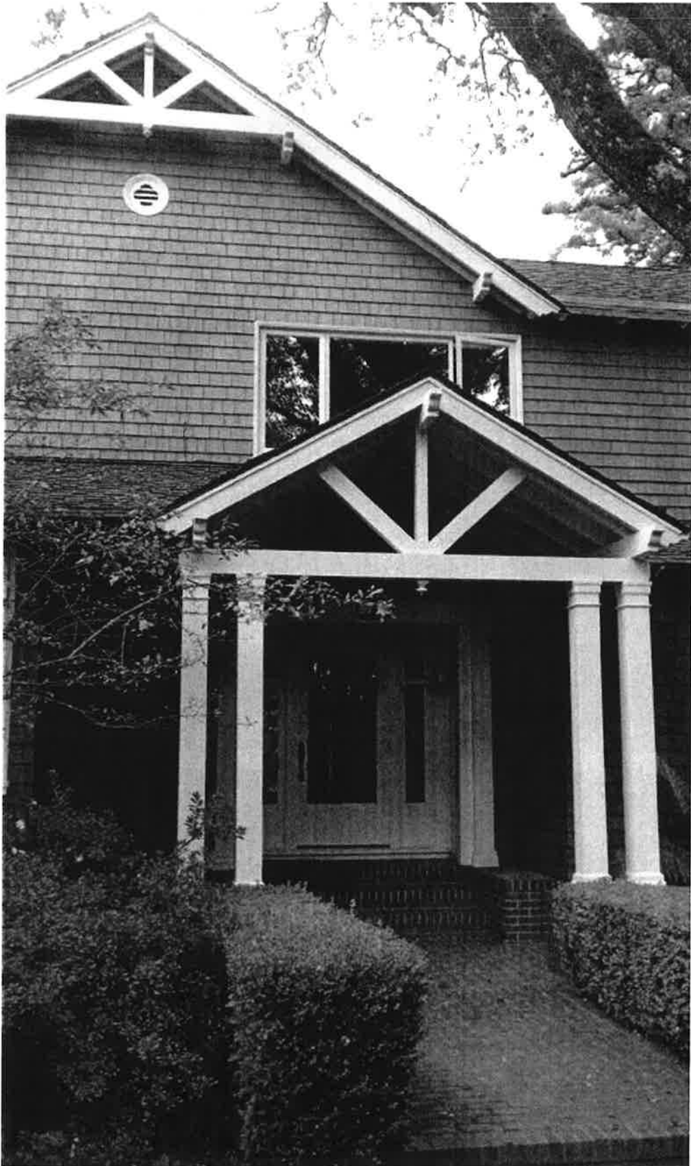
Fig.6 – 147 Lagunitas Rd. – Entry porch at east side (2014)
