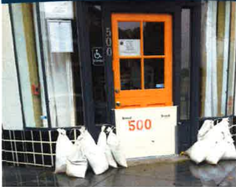
Merchants prepare for stormy weather by protecting storefronts with sandbags and floodgates.
