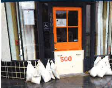
Merchants prepare for stormy weather by protecting storefronts with sandbags and floodgates.
