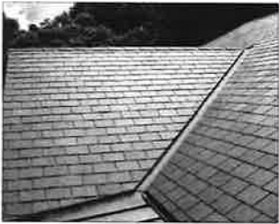
SLATE ROOF TME. D
