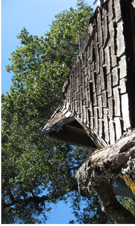
View 4. View of existing cabin on-site.
