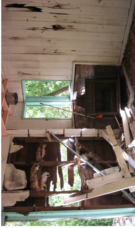
View 4. View of the interior of the existing cabin on-site.
