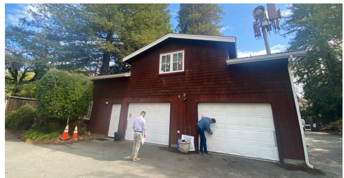
Public Works - Exterior
