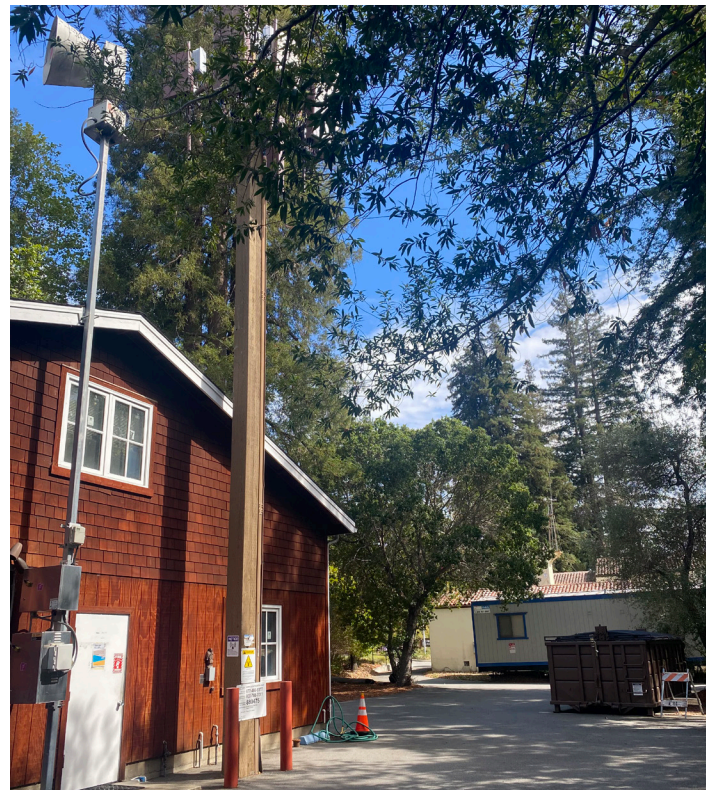
Public Works - Exterior
