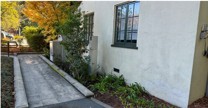
Town Hall - Exterior Ramp
