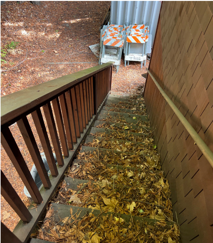
Public Works - Exterior
