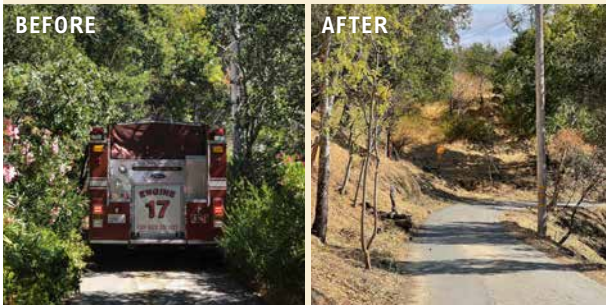
Evacuation Route Clearing in Greenbrae: Before and After
