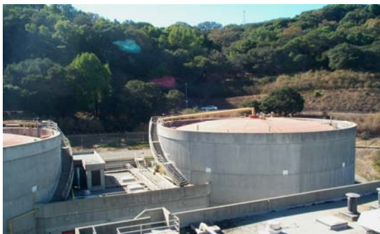
These existing CMSA anaerobic digesters would be used to convert food waste to methane gas .
