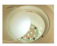
New technologies like this LED overhead light fixture can reduce energy use by as much as 80%.
