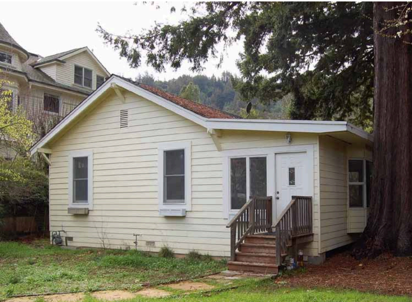
The Town's draft housing element provided for a number of affordable housing sites. The Council decided to remove the Town-owned property at 6 Redwood Drive from a list of potential multi-family housing sites and maintain the house as a single-family rental unit.
