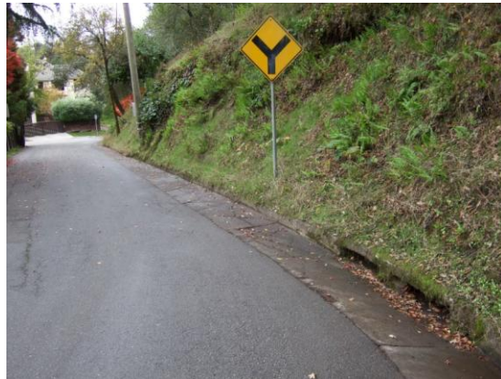
A view of a culvert inlet on Oak Avenue.
