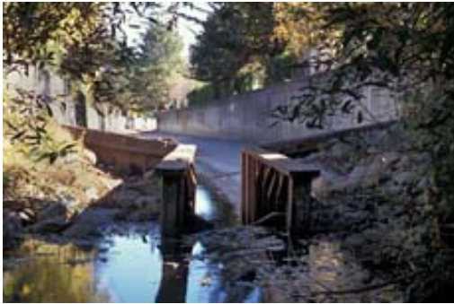
Existing fish ladder
